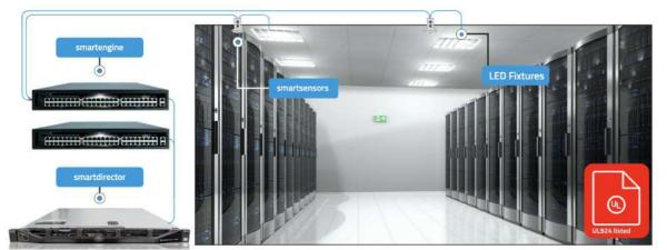
The smartdirector provides a browser based user interface for all of the smartengine devices, stores smartsensor data and provides web services and BACnet/IP APIs.
