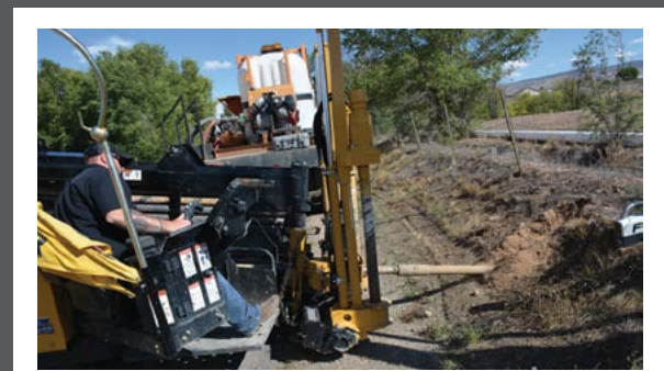
Directional boring and installing conduit for the underground fiber.
