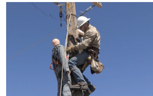
Pole-Top Rescue: A lineman safely brings an unconscious co-worker down from the pole top to ground level in order to begin CPR.
