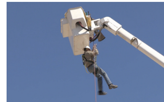
Fisk Descender: A lineman repels out of an inoperative bucket truck in order to save himself from a dangerous situation.
