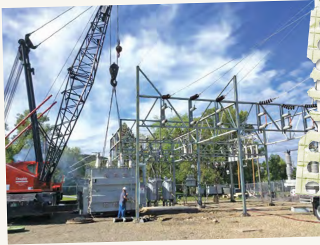
A CRANE LIFTS THE NEW PAONIA SUBSTATION TRANSFORMER INTO POSITION.
