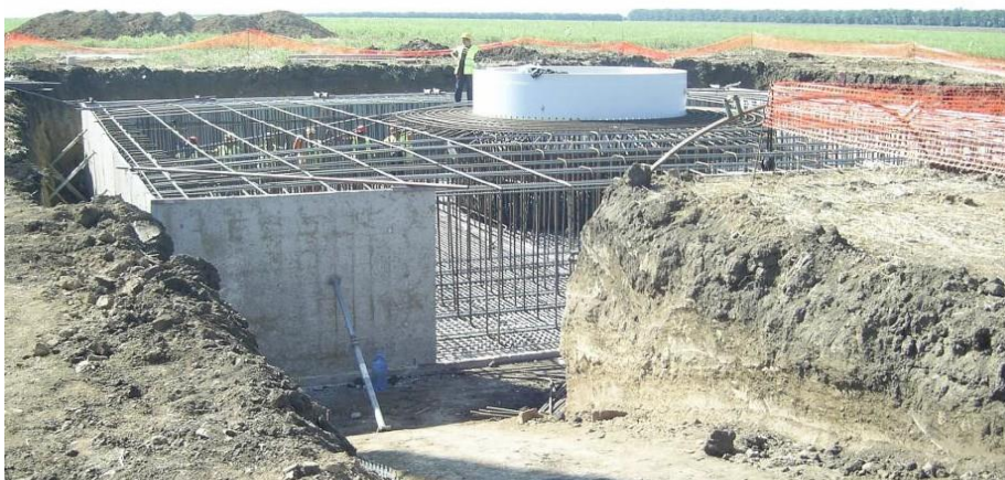
Figure 2.1-5. Formwork, concrete and reinforcement work on the wind turbine foundation
