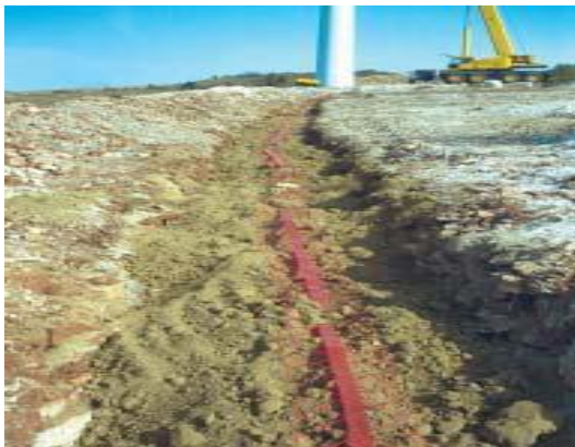
Figure 2.1-2. Trench for underground cables
