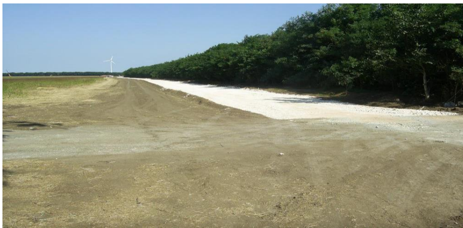
Figure 2.1-6. Graveling an existing country road
