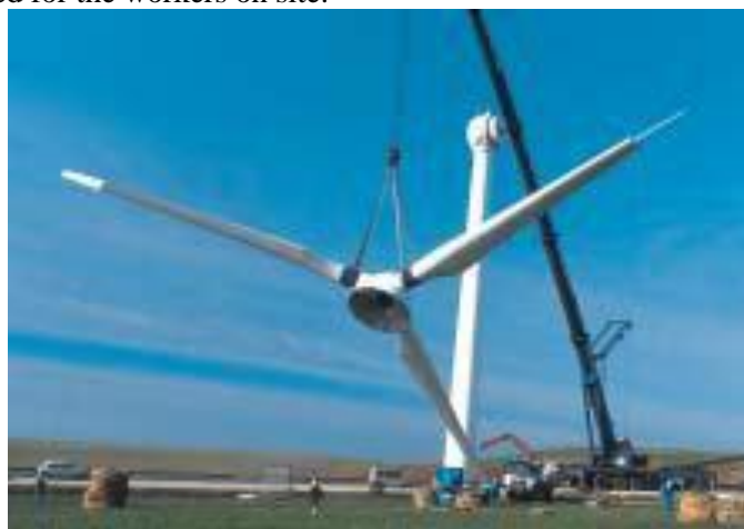
Figure 2.1. Rotor installation
