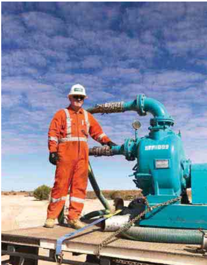
Pigging and cleaning activities, Gas flow lines, Moomba, South Australia
