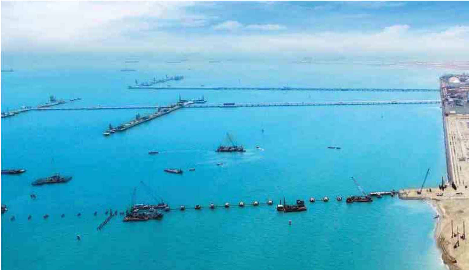
Pengerang Deepwater Terminals, Pengerang (Eastern View) – Phase 3 Development in progress
