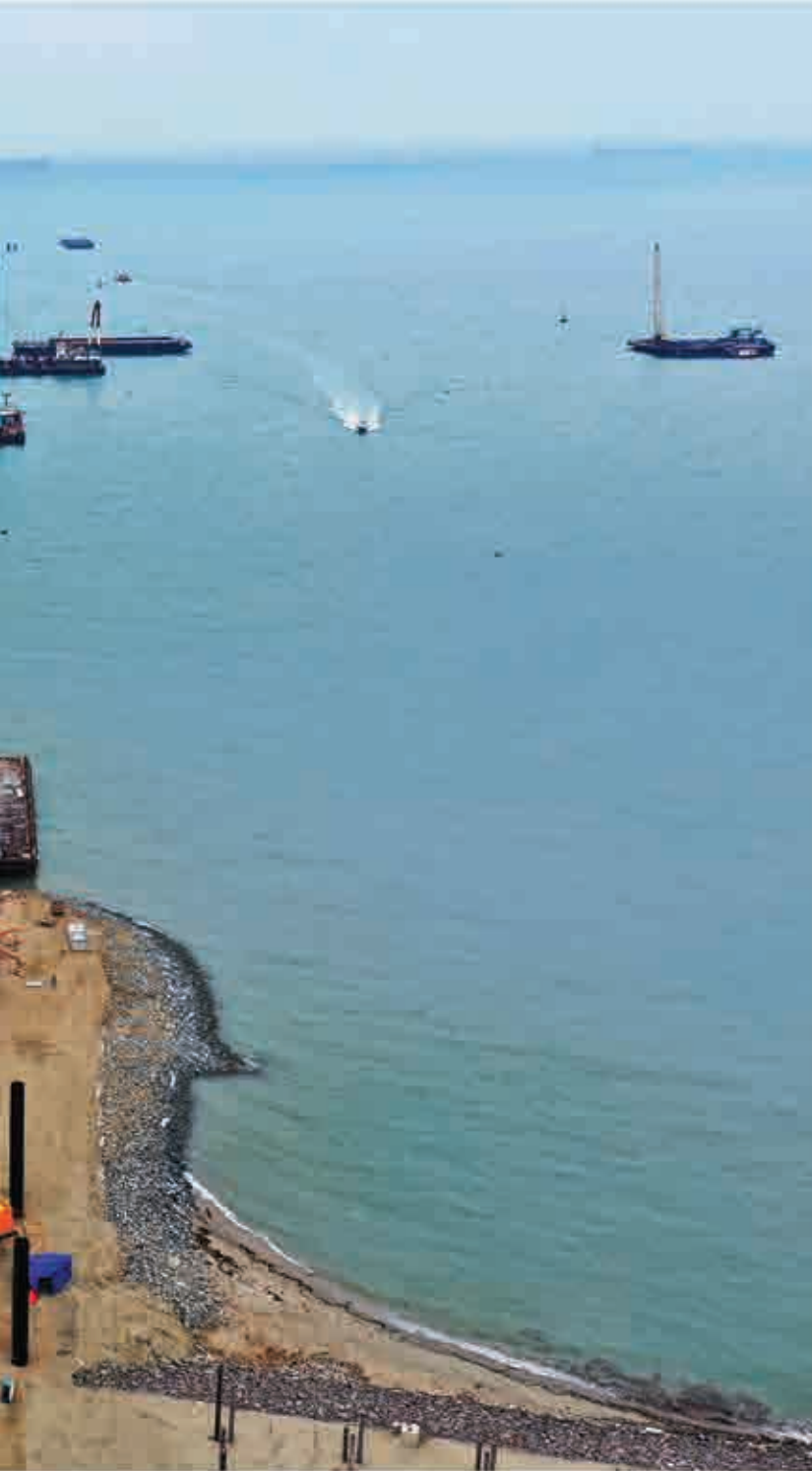
Piling work for Jetty 3, Pengerang Deepwater Terminals Phase 3
