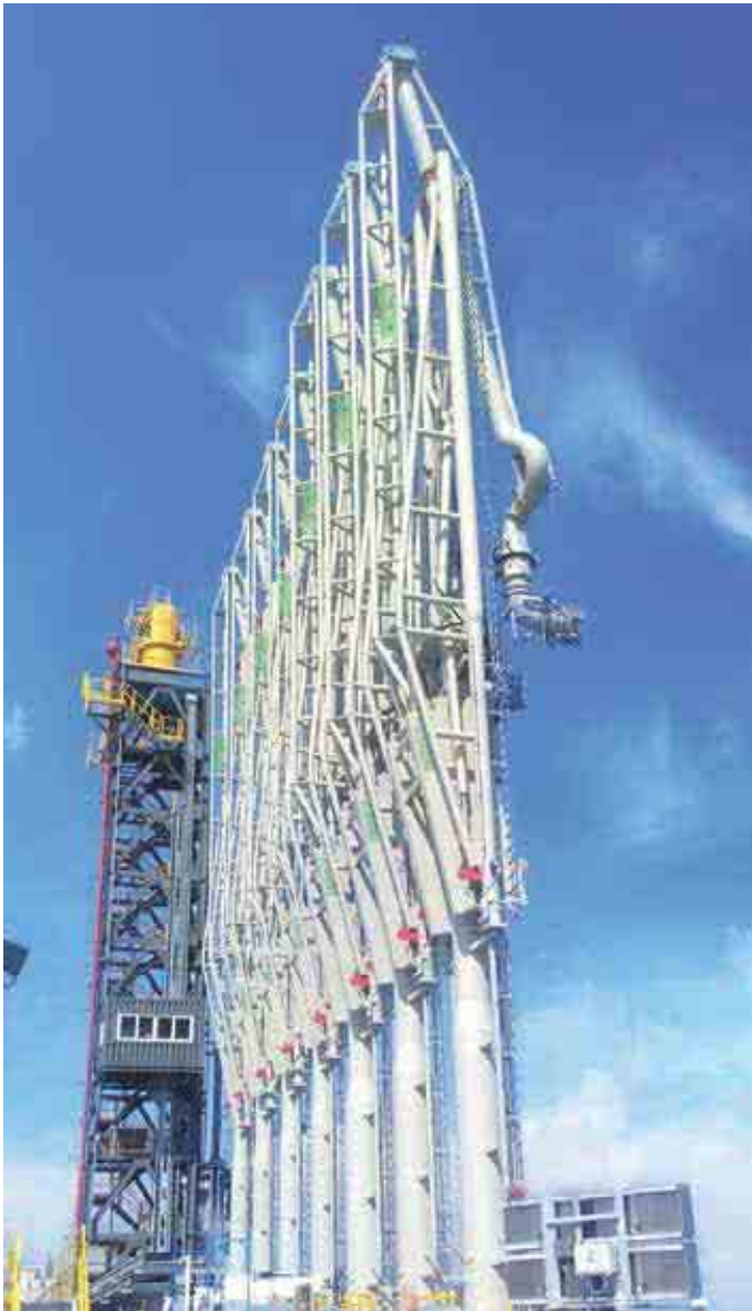
Marine Loading Arms at Jetty-2, Pengerang
