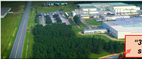
Meredian, Inc.'s sprawling 300,000 sq. ft. biopolymer manufacturing facility in Bainbridge, GA.
