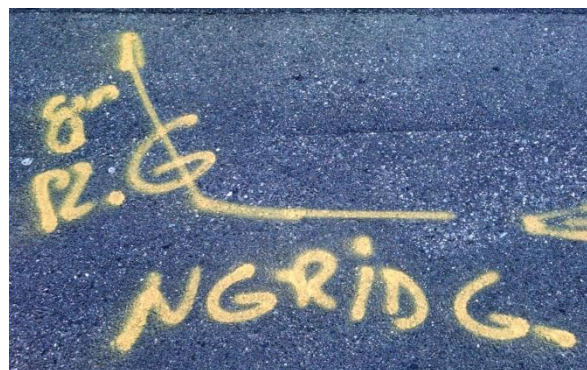
Figure 19. Gas Mark Out after Notifying Dig Safe
