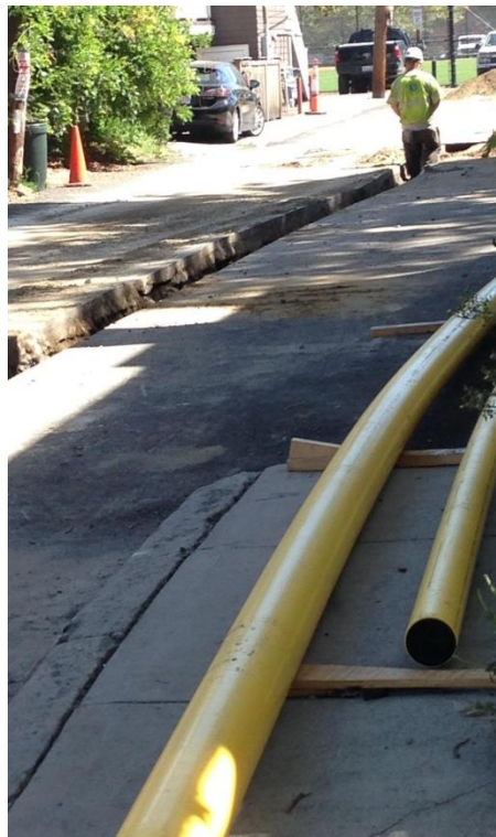
Figure 2. Plastic Gas Main Ready for Installation
