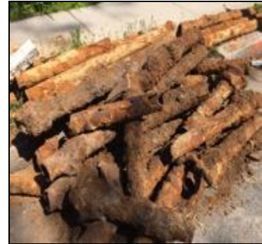
Old gas pipes
