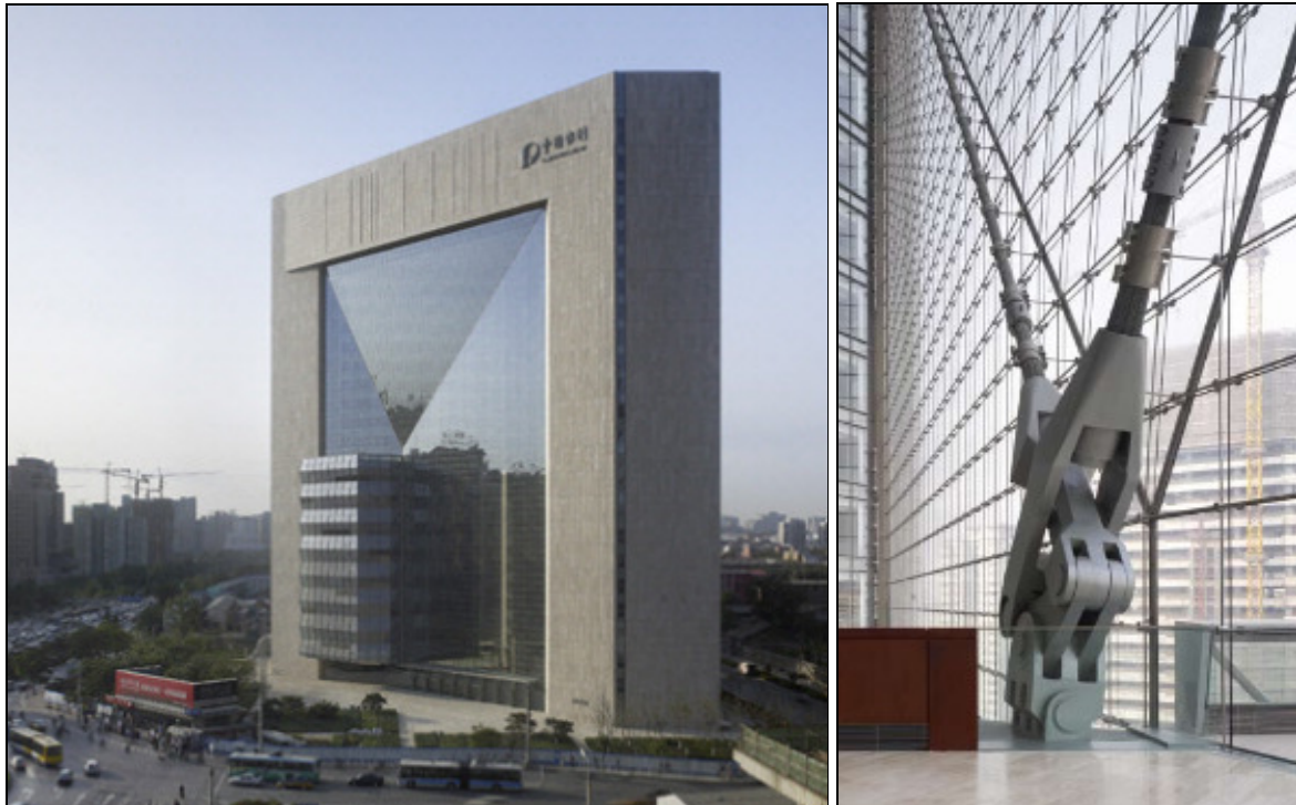
Figure 1. Casting use in Beijing Poly Plaza (photographs courtesy of Skidmore, Owings & Merrill LLP)
