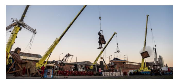
Given the show's fast pace, central location and audience size, Adlib decided to utilise large cranes to fly the audio systems so the appropriate amount of PA could be used for the larger scenes. This was a smart decision that also meant the same PA system could be used more than once in different locations over the course of the event.
