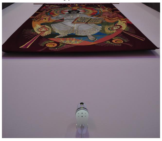
Though the rental system was ideal on a temporary basis, it was not suitable for permanent installation. The tripod-mounted camera was subject to movement or even theft; cables, though neatly run, could pose a hazard once the general public were readmitted; and the Web Presenter, though convenient, limited the resolution of the stream to 720p.
