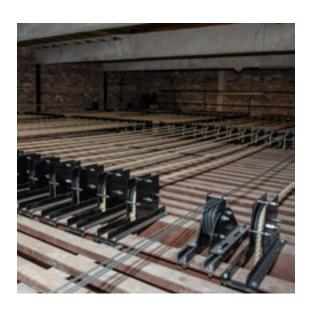
On the stage, electrically operated winch units raise and lower internally wired lighting bars. The rigging on stage was also enhanced by 32 new 3-line hemp sets with new pulleys, hauling ropes and suspension barrels.
