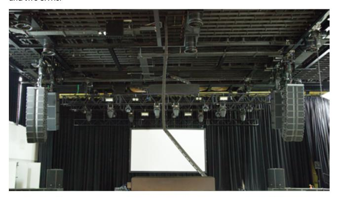
All the L-Acoustics elements are powered by proprietary LA8 and LA4X amplifiers and the Adlib speakers by Crown XTi 6002s. System processing is provided via a BSS Soundweb London BLU-160 networked processors.
