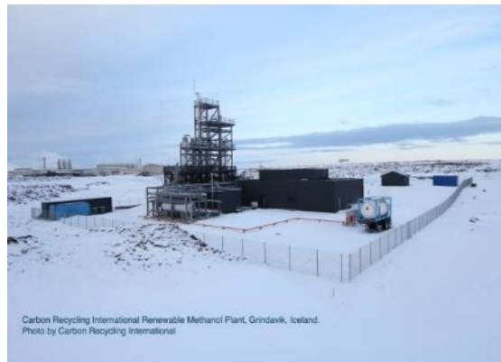
CRI's Power to Methanol plant, Iceland
