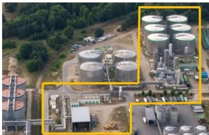
VERBIOgas plant in Schwedt, Germany
