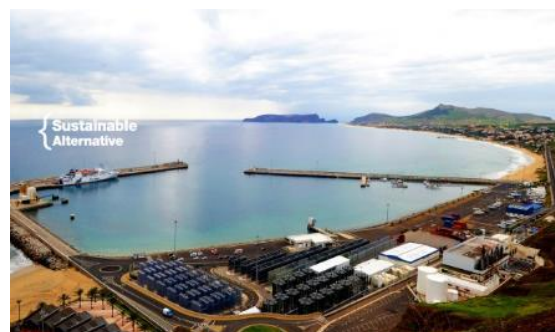
The Buggypower S.L. plant, Porto Santo, Portugal
