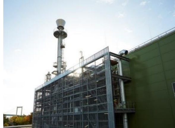
GoBiGas plant in Gothenburg, Sweden
