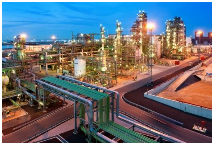
Neste's HVO plant, Rotterdam, The Netherlands
