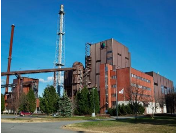
Fortum's plant in Joensuu , Finland
