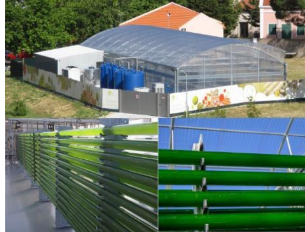
Overview of A4F Lisbon Experimental Unit and tubular photobioreactor of 1,000 L – Designed and built by A4F. (DEMA FP7 project)
