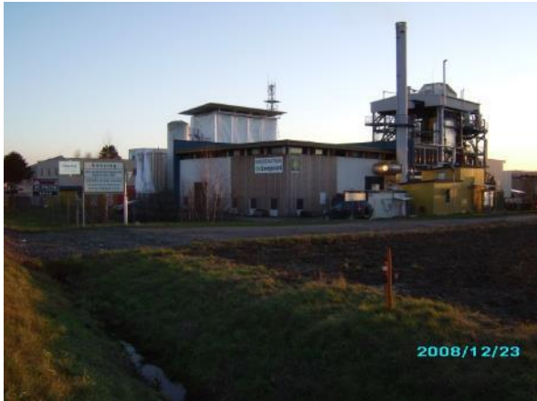
Biomass CHP Güssing, Austria
