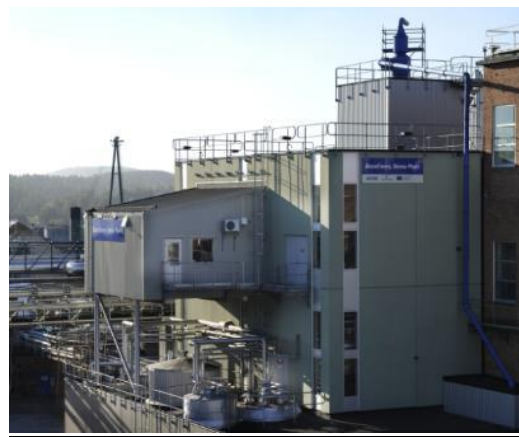
The SEKAB Plant, Sweden
