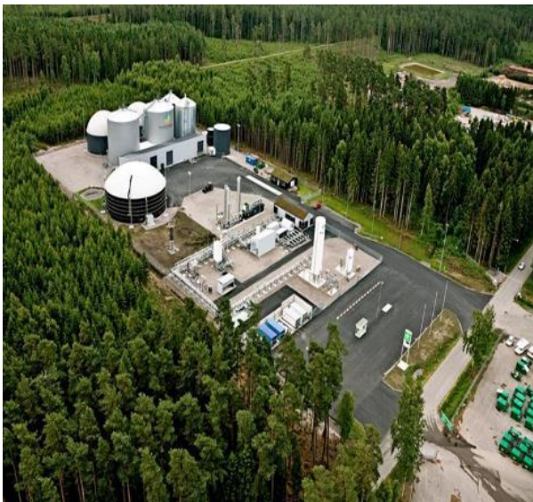
Lidköping Biogas - Air Liquide and Swedish Biogas International in Lidköping, Sweden
