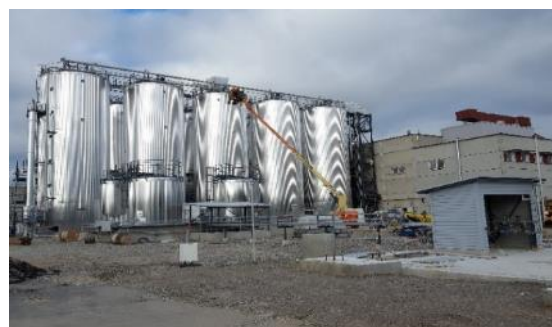
Cellunolix® plant under construction, Kajaani, Finland
