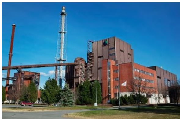
Photo 9 Fortum's Joensuu plant in Finland
