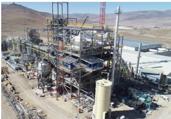
Photo 8 The TRI plant under construction at Reno Nevada, USA
