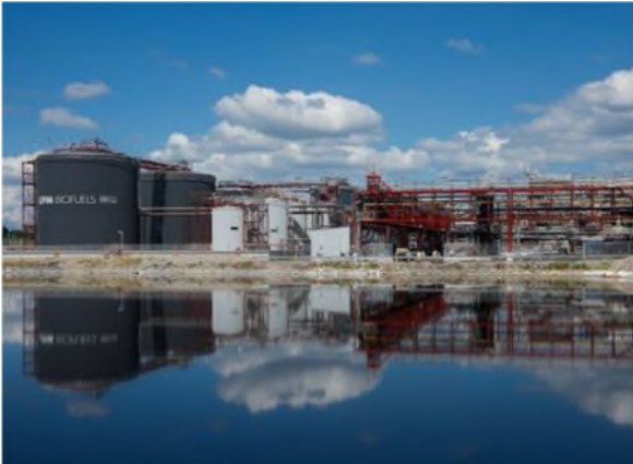
Photo 15 UPM's Lappeenranta biorefinery plant
