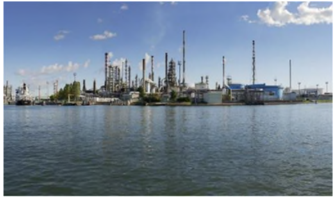
Photo 14 ENI's Green Refinery plant in Venice
