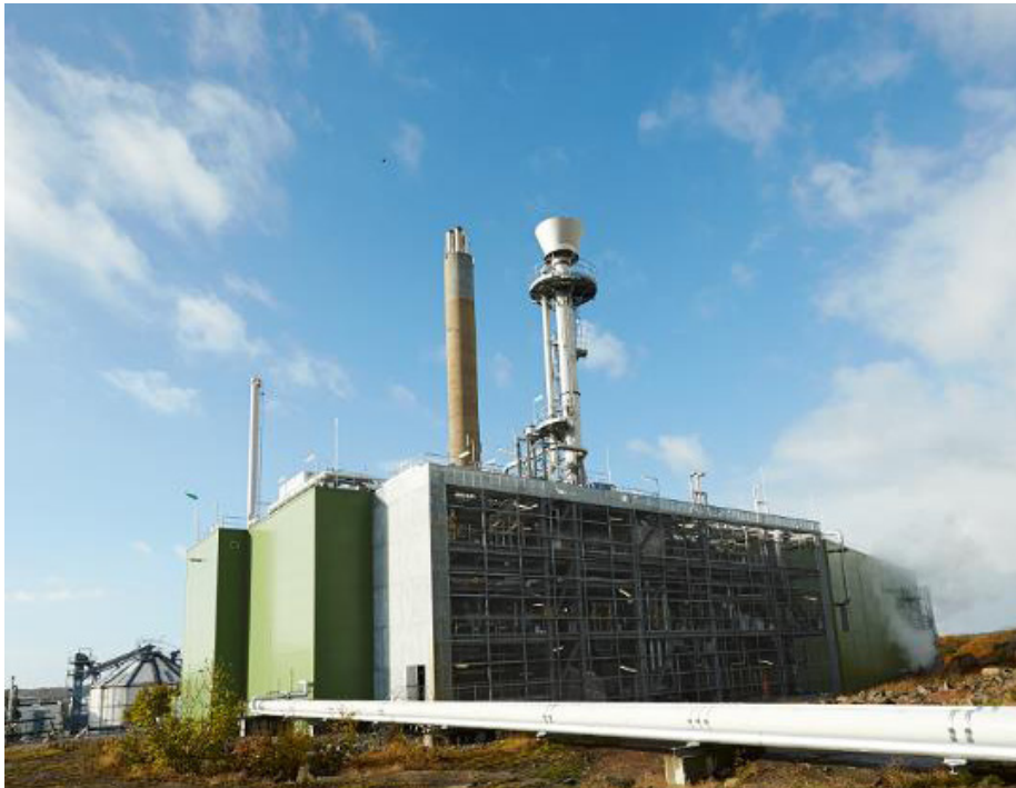
Figure 4.1 The GoBiGas plant in Gothenburg is the first of its kind in the world, injecting biomethane from thermal gasification and methanation to the natural gas grid of Gothenburg. At full production, the 20 MW methane plant will deliver 160 GWh/yr. (Photo: Used with permission of Rob Vanstone and Göteborg Energi, Sweden).
