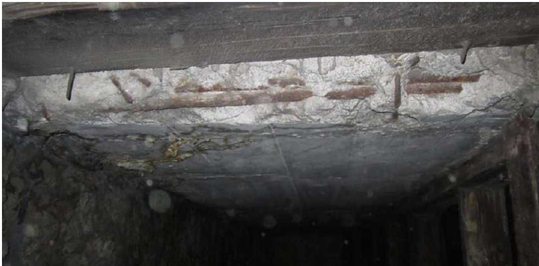
Figur 5-8 Armeringskorrosion (Ri.se, 2019)
