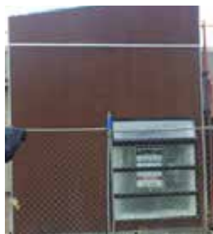
0 MONTHS: Recently built, this shows the beginning colour of Weathertex Natural boards.
