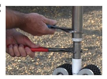
Remove the 3/4" stainless rod from the topmost sucker rod (left). To remove the 3/4" stainless rod without damaging it, attach your channel lock (or vice grips) to its flat section, at its top.
