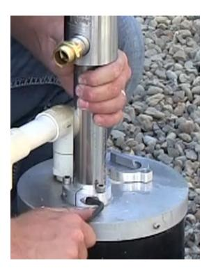
Using the 1/4" Allen wrench, loosen the pinch bolt and the 3 mounting bolts on the split flange (left) enough to pull the pump head (including riser tube) up out of the well.
