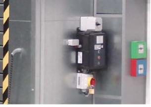
In normal operation, the roller shutter opens and closes using the buttons on the control unit by impulse activation.
