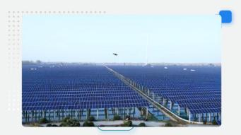
The drones can be programmed to autonomously take off from their docks at a scheduled time, follow specific flight paths, capturing images of the solar panels from different angles. The images are then analyzed using Al algorithms to identify any faults or issues, such as damaged panels or vegetation growth. This information is relayed in real time to maintenance teams, who can then prioritize their efforts accordingly.
