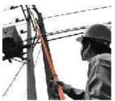
Our fabricated Disconnecting sticks are capable to withstand voltage up to 250 kV and up to 400 times aging. In addition to regular production of disconnecting sticks, we also going to introduce telescopic disconnecting sticks to save the storage space and give even easier move.
