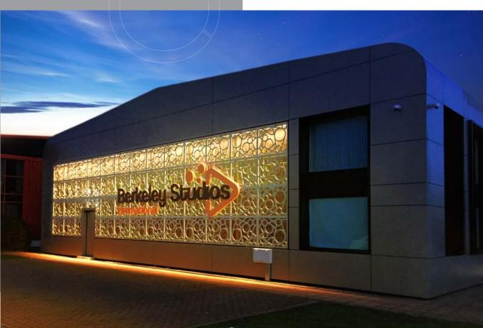
The project consisted of an entire over haul of the existing façade with the introduction of a new vitra bond cladding system, new windows throughout and new guttering system. Importantly, all works were carried out while the occupants still maintained full production capability.
