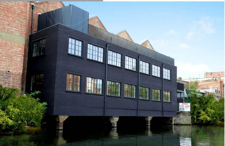
We carried out the strip out and Cat A refurbishment of 25B Vyner Street. The project was logistically challenging as it sits right up against the Regent's Canal. The original plan was to set up a cantilever scaffold system at the rear of the building which would have taken up window and floor space on the ground and first floor.
