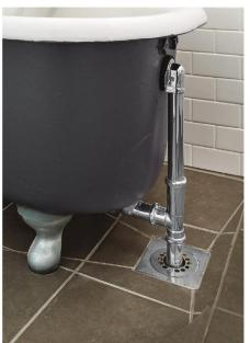
A shower pan and drain under the tub catches overspray from the shower, which is curtained off, floor to ceiling, outside the soaker.
