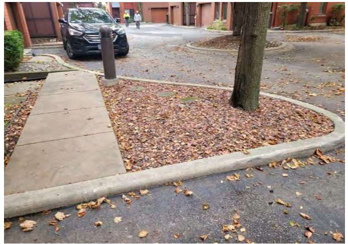
Overview of concrete curb
