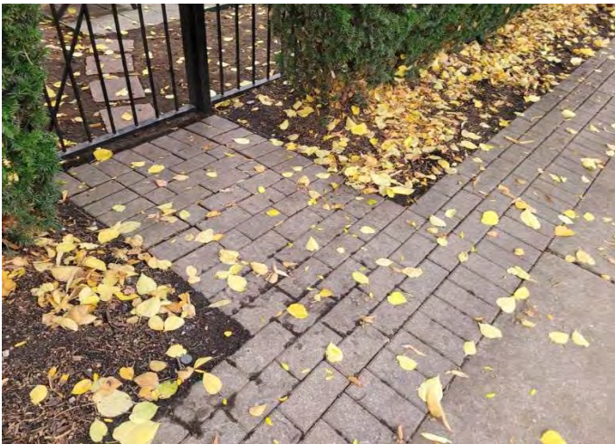
Pavers along public walkway and leading to unit gate
