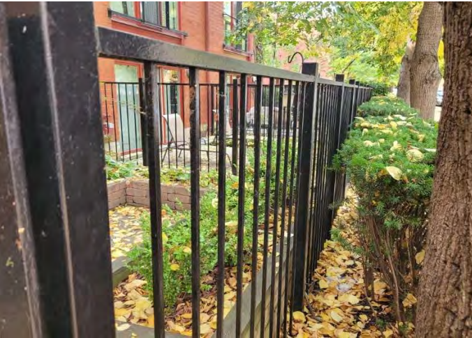
Overview of fencing at enclosed unit yards
