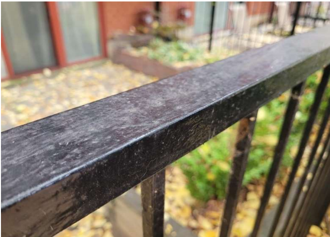
Paint finishes at fence rail and pickets
