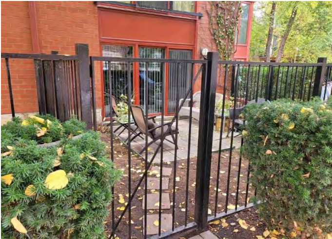
Metal fencing and gate at unit yard
