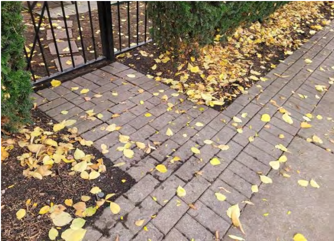
Pavers along public walkway and leading to unit gate
