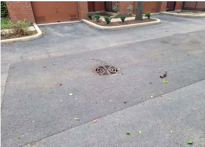
Catch basin with replaced pavement surround
