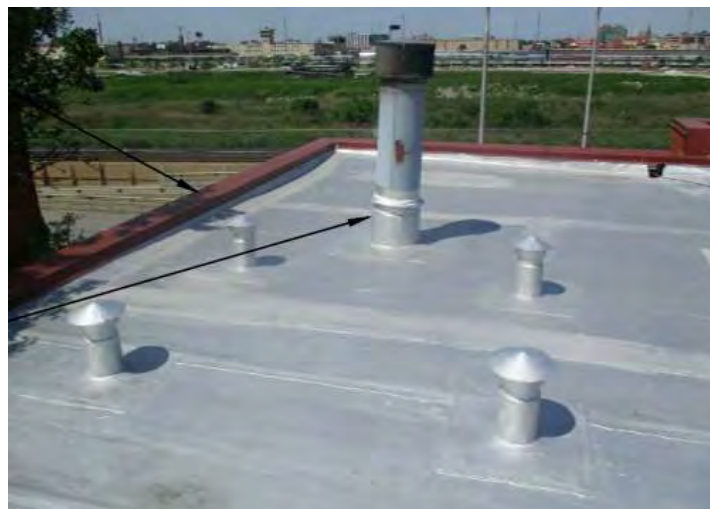
Existing roof not yet replaced
