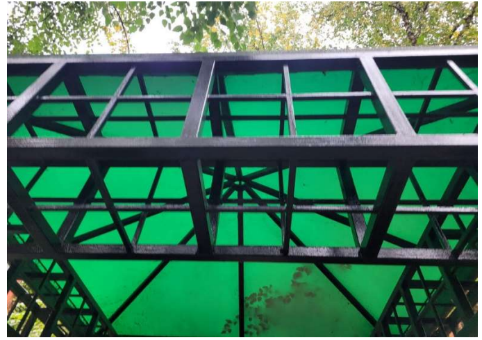
Painted steel frame at gazebo
