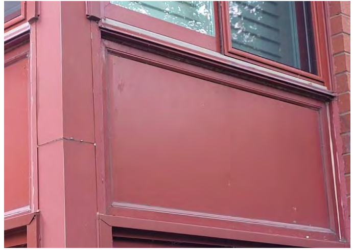
Metal window spandrel panels and corner trim
