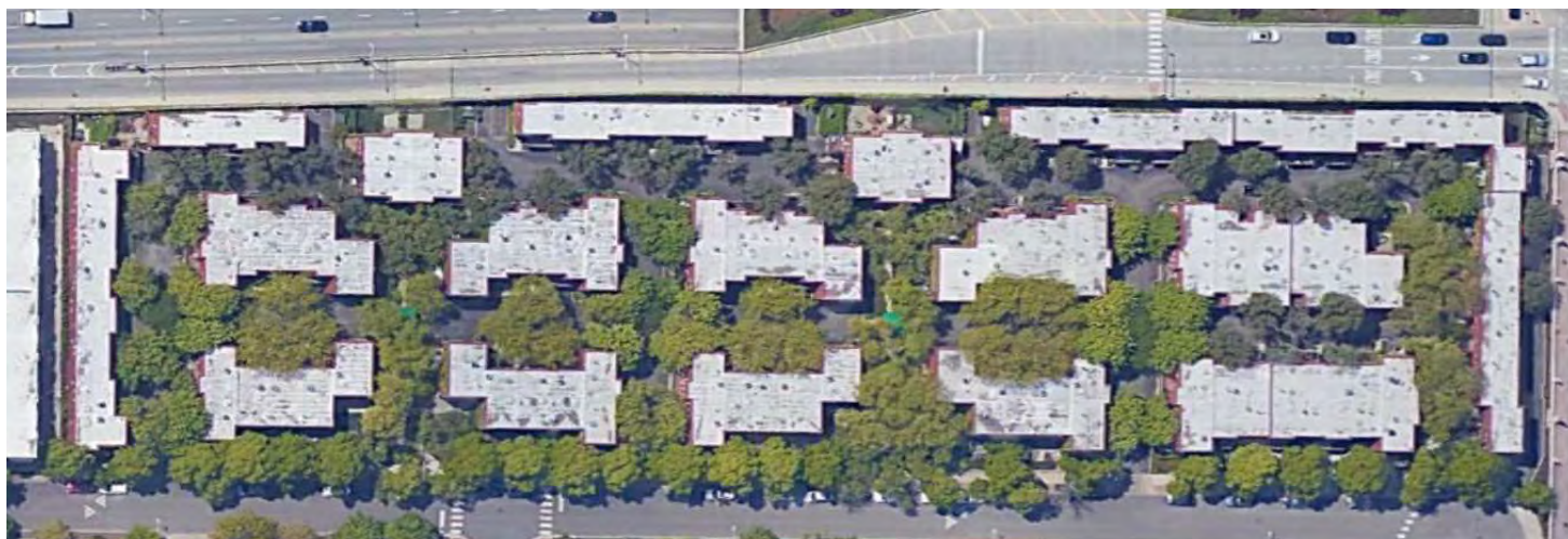
Aerial view of flat roofs
