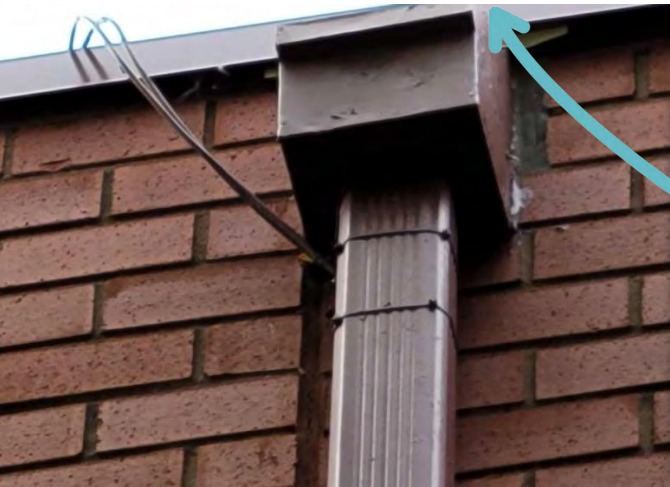
Aluminum scupper box and downspout
