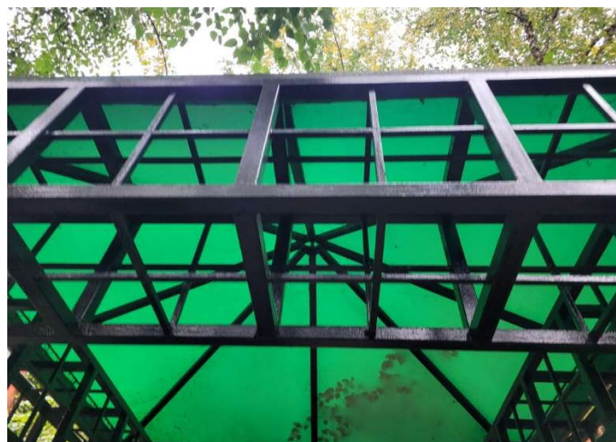
Steel frame at gazebo
