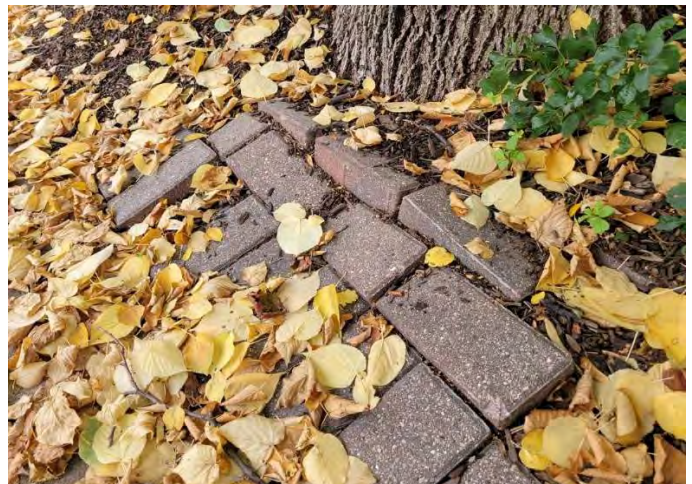
Unlevel paver surface adjacent to tree roots
