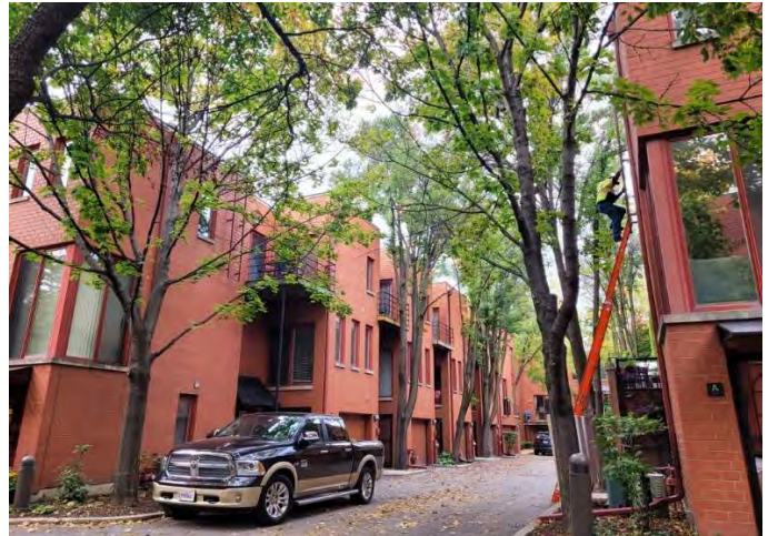
Mature trees in close proximity to buildings
