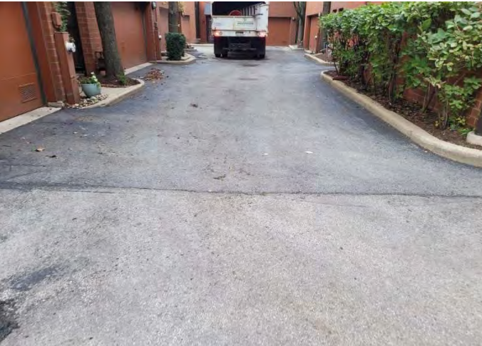
Overview of asphalt pavement
