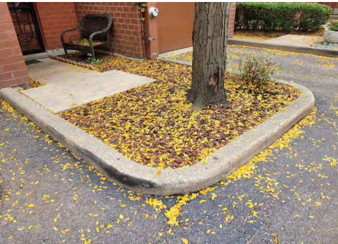
Overview of concrete curb
