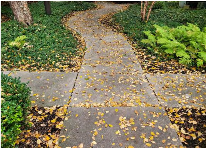
Overview of concrete sidewalks at common area
