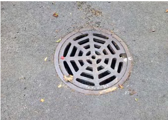
Catch basin at pavement
