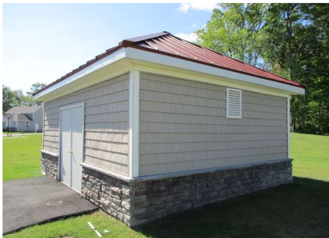
Existing BLN well house
