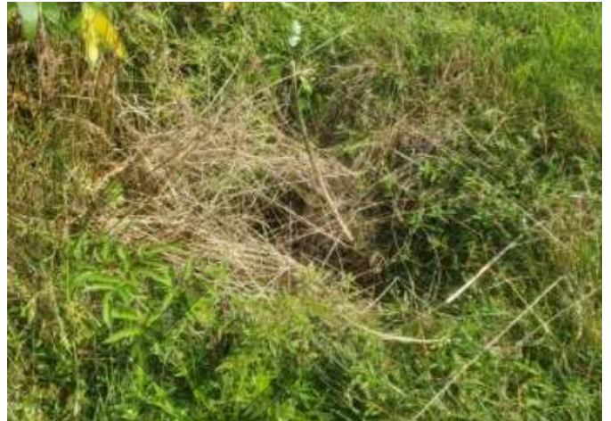
Rill formed at Pond #3 behind lot #401 - photo from Envirotech report
