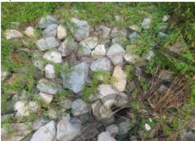
Final outfalls with vegetation growth - photo from Envirotech report.
