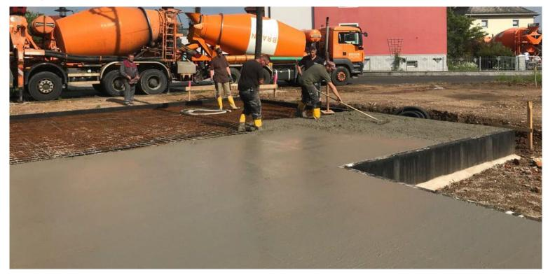
After compaction, a separating layer is applied, reinforcement is laid, and the standard concrete works are carried out. Info: solid wood ceiling elements are often being installed to save on concrete.
