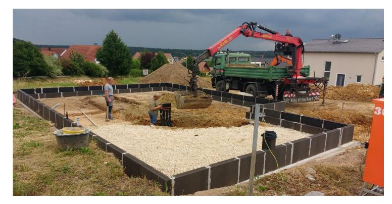
Assembly of formwork "RDS" (Randdämmschalung) elements using GLAPOR boards - eliminating wooden formwork and subsequent end-face insulation work.
