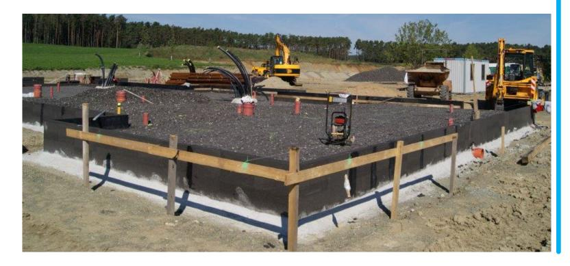
The GLAPOR cellular glass gravel is distributed loosely using a rake and subsequently compacted with a standard vibrating plate. Just like sand.
