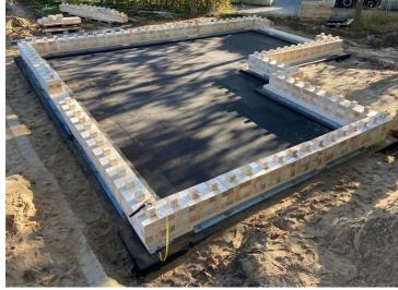
Berlin 10/23: Worldwide first concretefree foundation and floorslabs: Floor, Insulation and Waterproofing in ONE section. Fully reusable.
