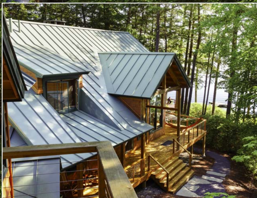
Wraparound porches and decks built of red cedar surround the cabin and garage.
