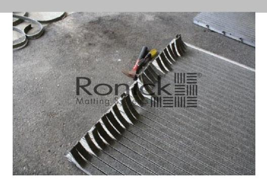
Existing carpet inserts are fastened down by rivets. To break rivets use hammer and chisel.
