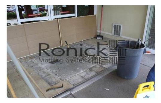
Remodeling begins by removing the tiles around the parameter.
