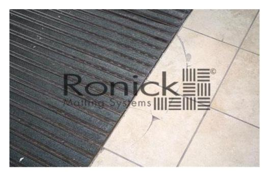
High Pedestrian traffic as well as ice melt and sand weakened the tile causing it to crack.
