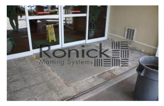
The existing thin set/mortar needs to be removed. This can be done with a bead blaster or a grinder.
