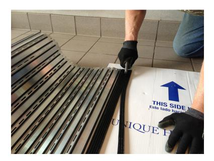
This filler is provided so that you can do an on-site custom fitting of your new mat. As illustrated, the filler can be easily cut using a razor and a straight edge, ensuring a snug, custom fit
