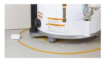
Alert Labs smart water leak sensors guard against water damage in key areas.
