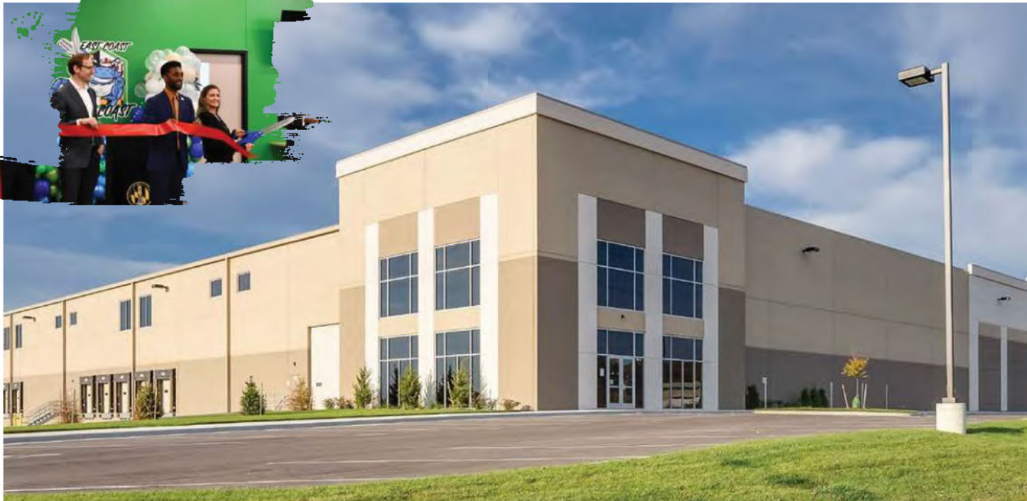
Harbor Logistics Center
