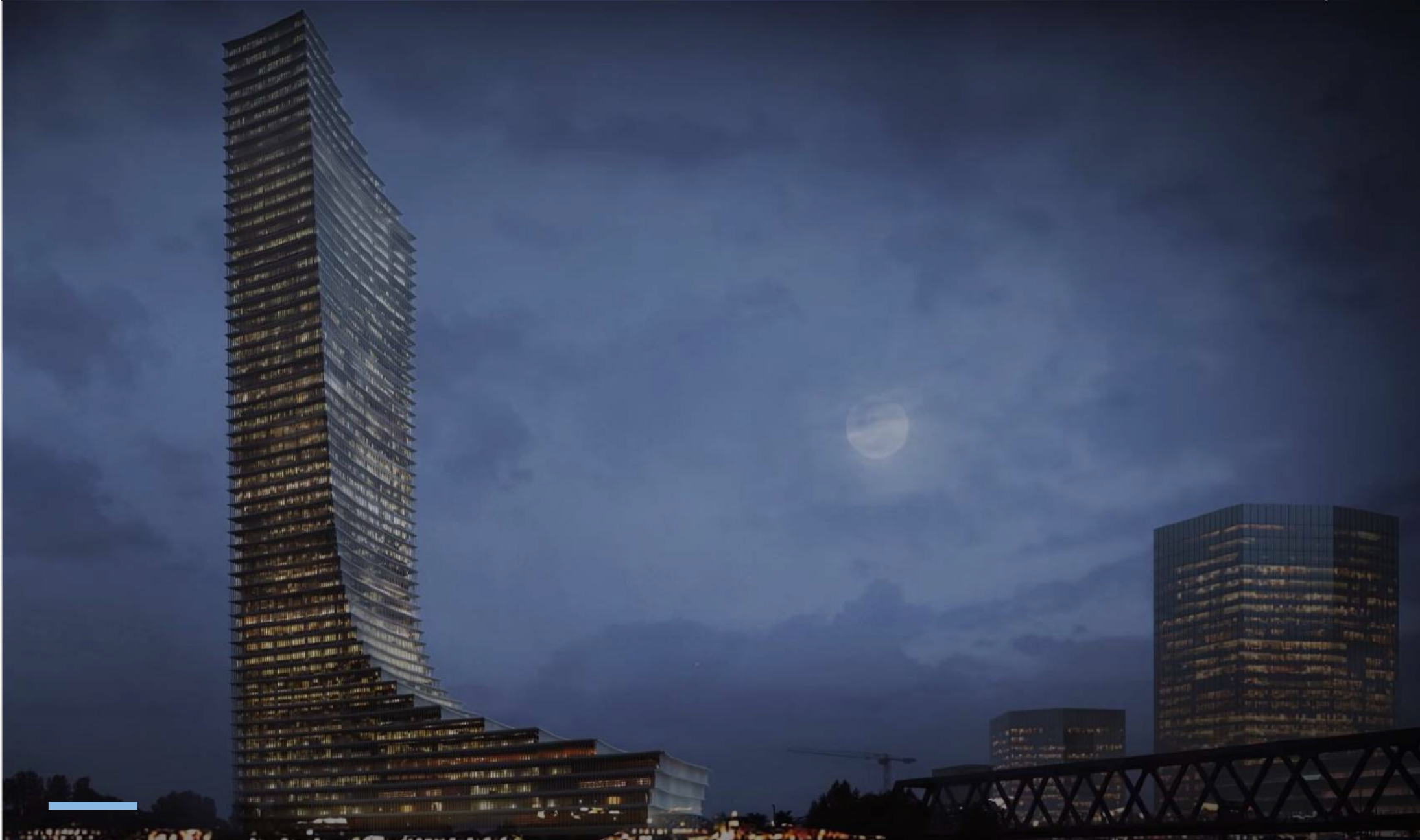
Hamburg | ElbTower, 254 mt, Commercial | TECMA Digital Platform Technology
