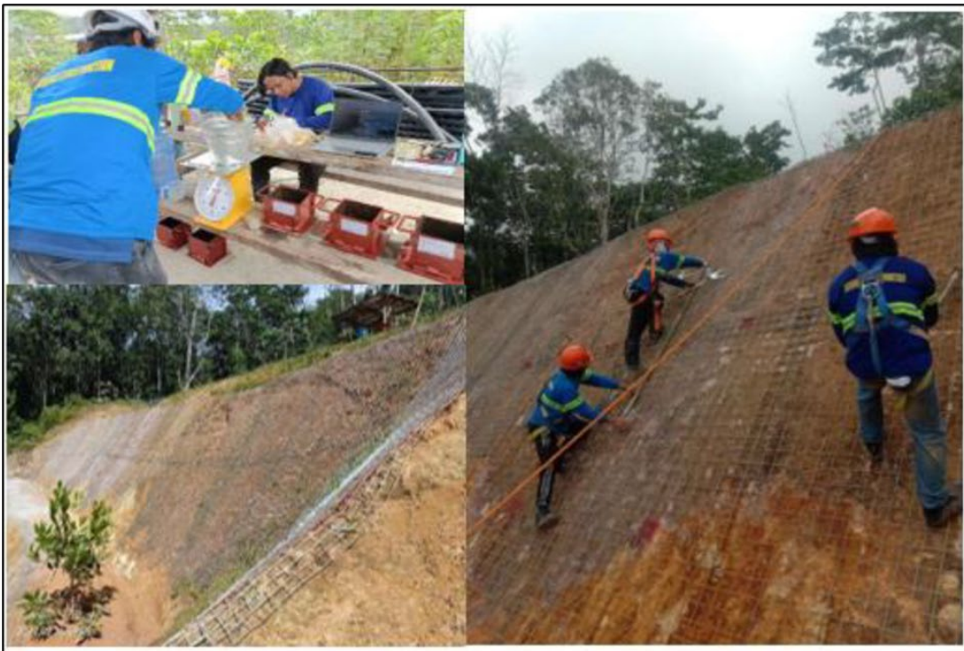
Photo 1: Wiremesh Installation at the Portal Slope
