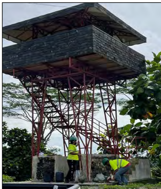
Photo 31. Upcycling of safety boots and used HDPE pipes as roofing and walling of view.
