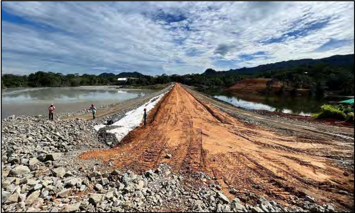
Photo 1. Ongoing construction extension of TSF#5B. Crest view.
