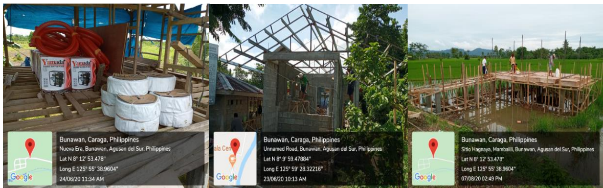
Picture 3. Water Pump Rentals for Water Refilling Stations of Brgy. Poblacion and Brgy. Mambalili, Farmers Association
