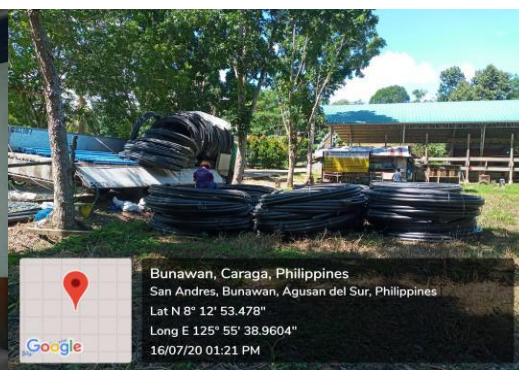
Picture 7. Pipelines (PE HOSE) water system of Brgy. San NDRES, BADS
