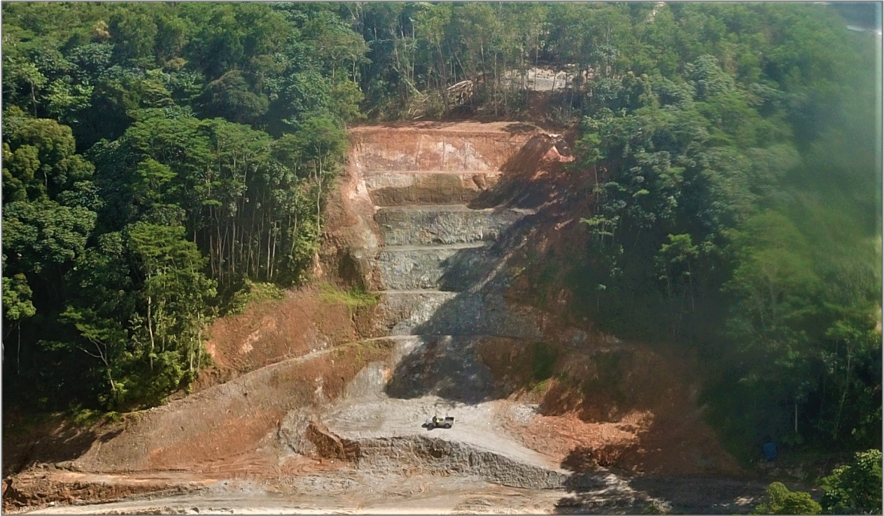
Photo 1: View of the portal area for the Tigerway Decline Portal.
