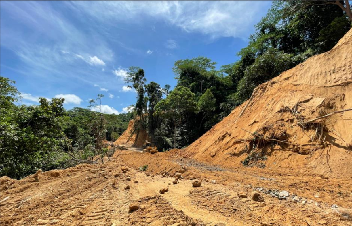
Photo 2. Ongoing extension of the water diversion canal.
