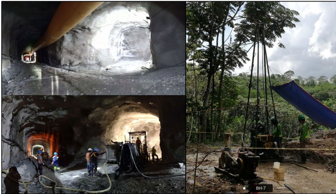
Photo 1: (Left) Tigerway substation excavation; (Right) Surface Geotech drilling
