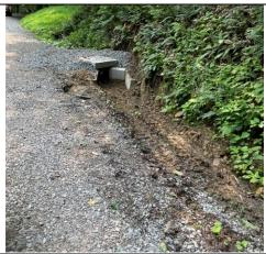
**Practices Used:** 7 new cross pipes, 4 replaced cross pipes, 1,620 tons road fill, 500 ft underdrain, 300 ft select thinning, 67 sq yd seed/mulch
