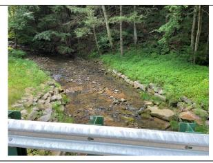
**Practices Used:** 4 new cross pipes, 336 tons road fill, 2 in-stream stabilization structures (J-hooks), 27' spread footing bridge
