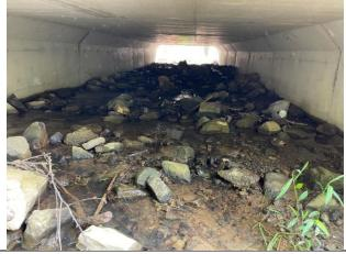
**Practices Used**: (site length: 354 ft) stream crossing replacement: new 10' box culvert with bottom, 5 instream stabilization structures, 1 other practice (demo of upstream obstruction)
