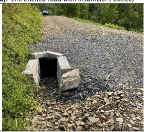
Practices Used: (site length 763 ft) 6 new cross pipes, 2,200 tons slate fill (605' x 24' x 2'), 440 tons DSA
