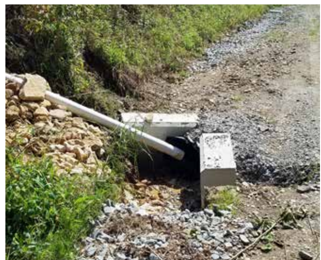
(After) A newly installed pipe to catch field drain
