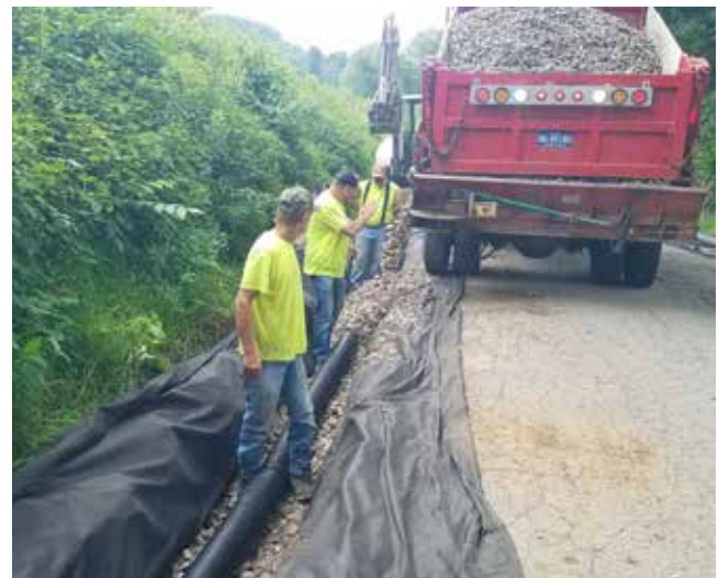
(During) Installation of underdrain
