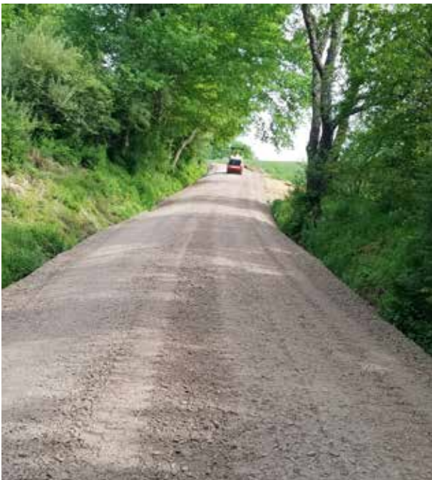
Adding limestone fill material
