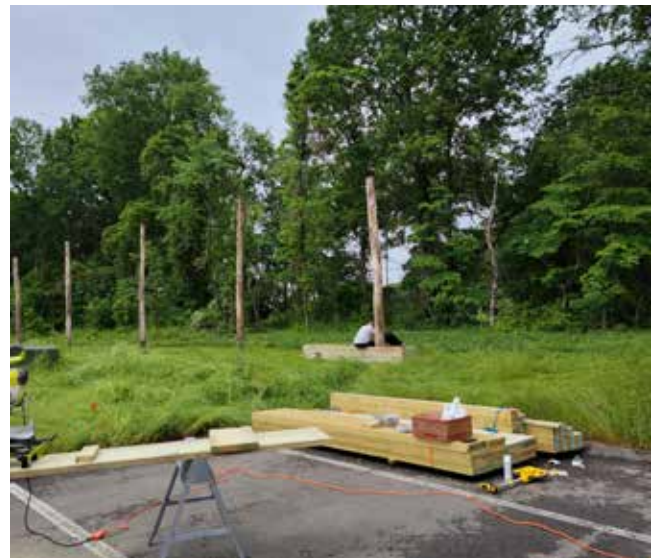
Installing growing poles
