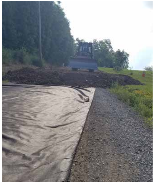
(During) Raising road profile with slate fill
