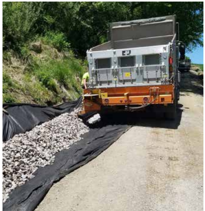
Installation of underdrain
