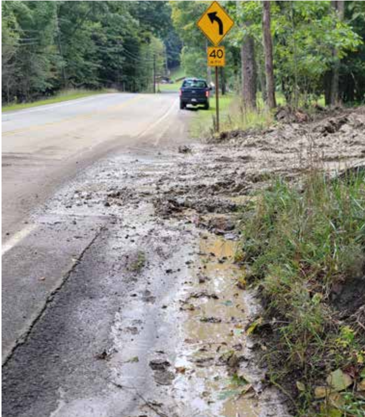
Active pollution from timber harvest site that did not have erosion and sedimentation control measures installed
