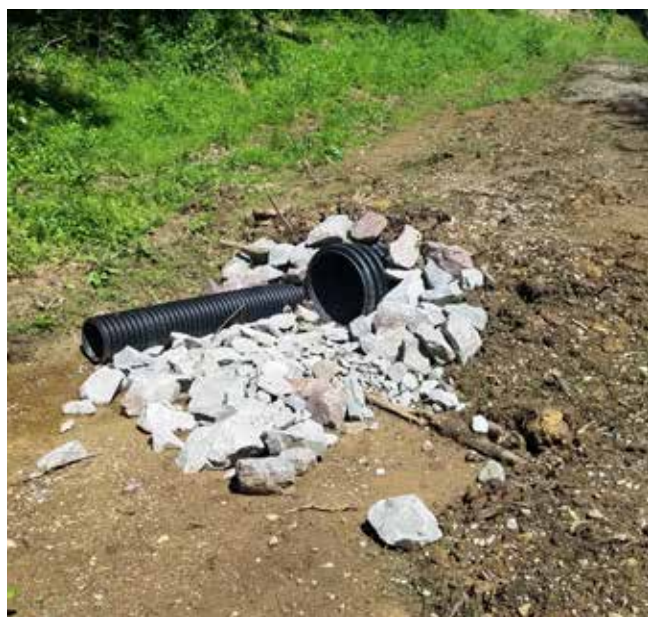
Newly installed stormwater pipe and underdrain outlet
