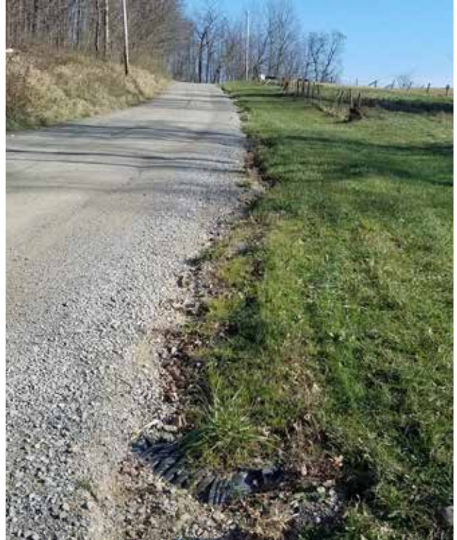
(Before) Entrenched roadway
