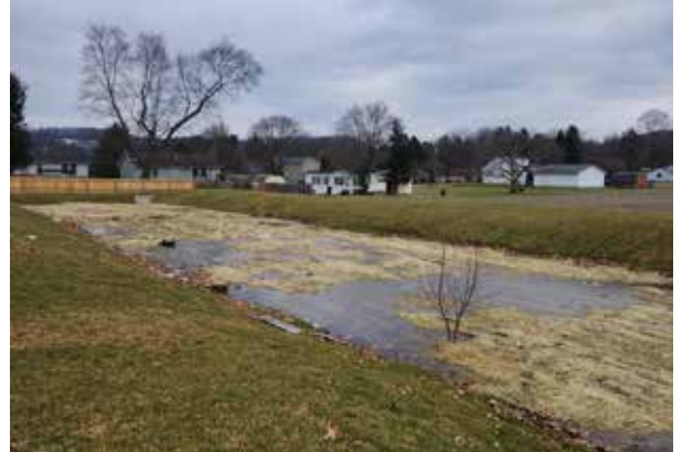
Non-functioning Rain Garden
