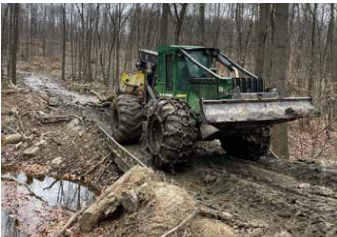
Unpermitted stream crossing that was installed correctly
