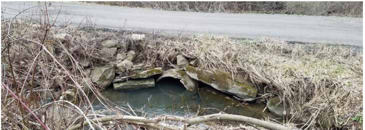
Before installing stream crossing
