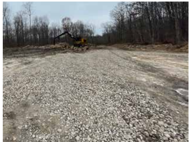
Rock Construction Entrance
