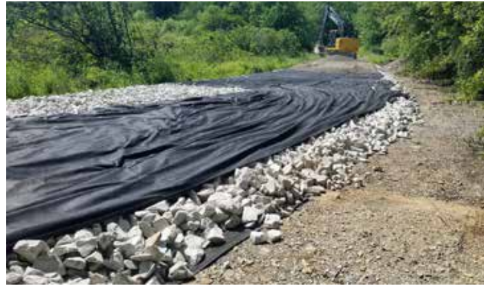
Installing french mattress
