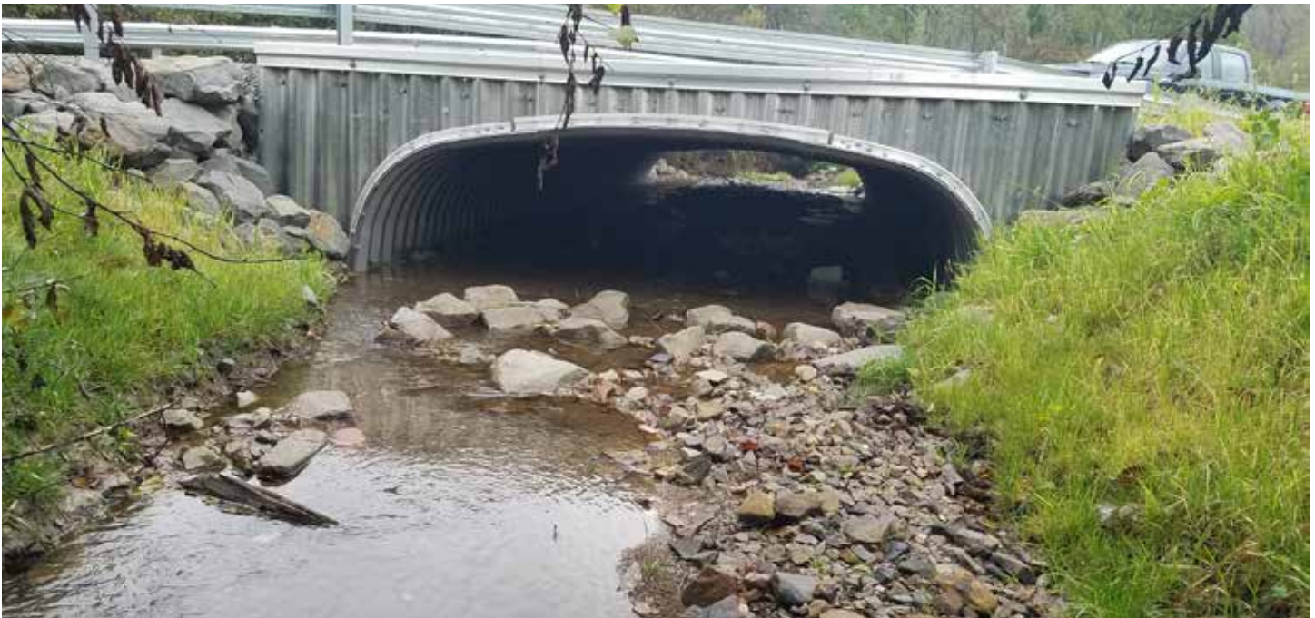
After installing stream crossing
