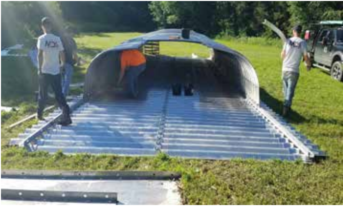
Building the stream pipe
