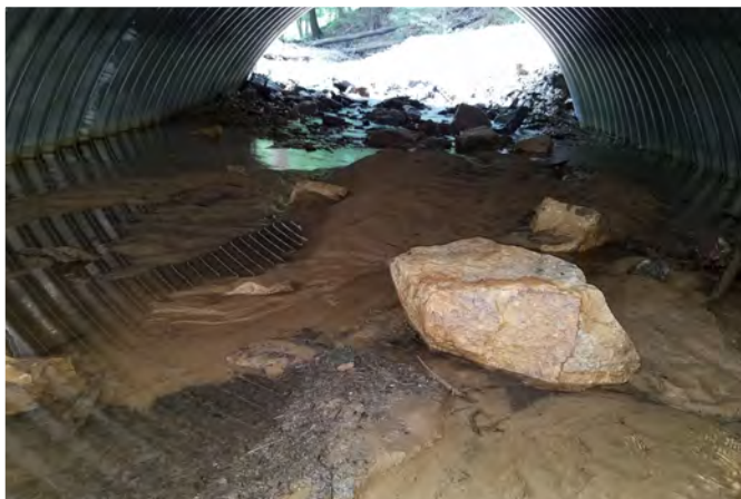
Left—Streambed material inside the newly installed culvert. This not only extends the life of the aluminum by preventing abrasion, but it also mimics a natural stream to allow aquatic species to move through the pipe and access upstream habitat.
