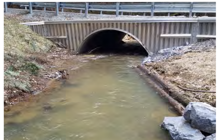
Left—Streambed material inside the newly installed culvert. This not only extends the life of the aluminum by preventing abrasion, but it also mimics a natural stream to allow aquatic species to move through the pipe and access upstream habitat.
