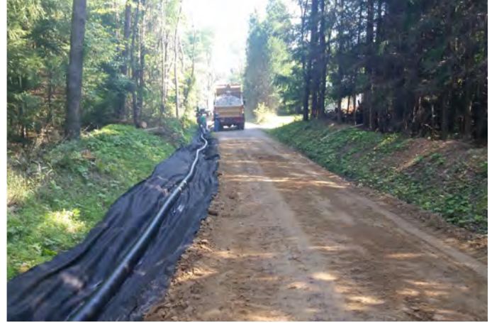
Active construction during road fill, left, underdrain installation, right.
