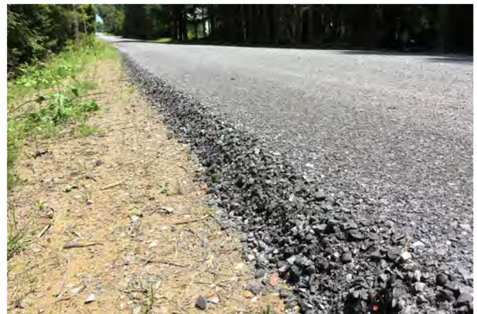
Driving Surface Aggregate was paver-placed as a final driving surface following drainage work.
