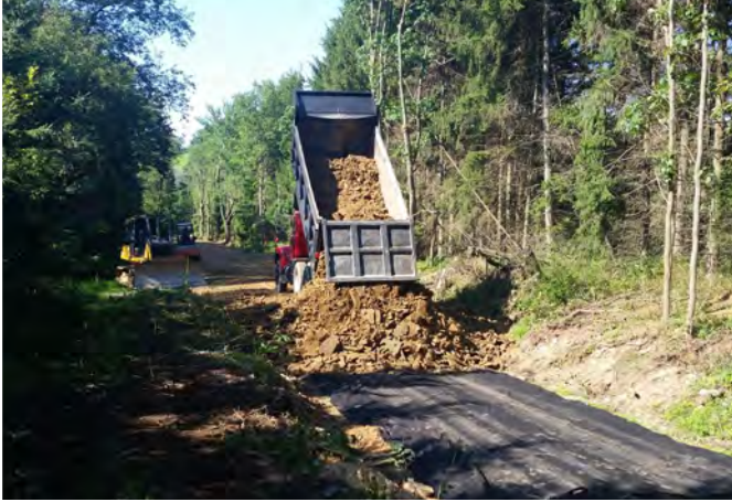
Active construction during road fill, left, underdrain installation, right.
