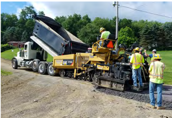
Driving Surface Aggregate was paver-placed as a final driving surface following drainage work.
