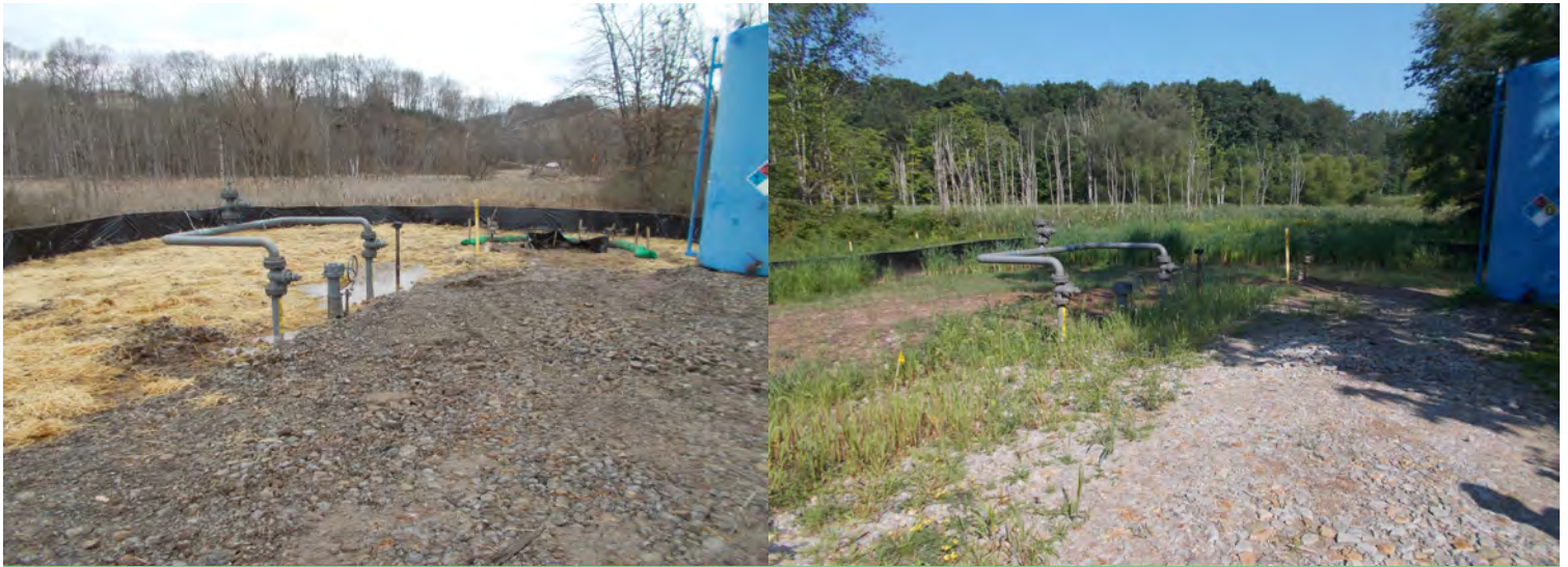
Before and after of pipeline restoration
