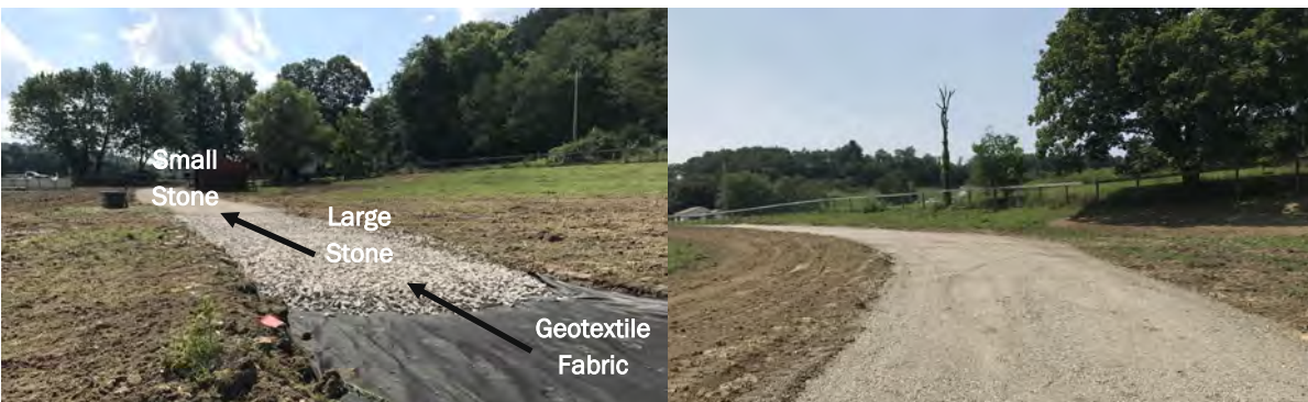
Installation of gravel animal trails on the Gromley Farm
