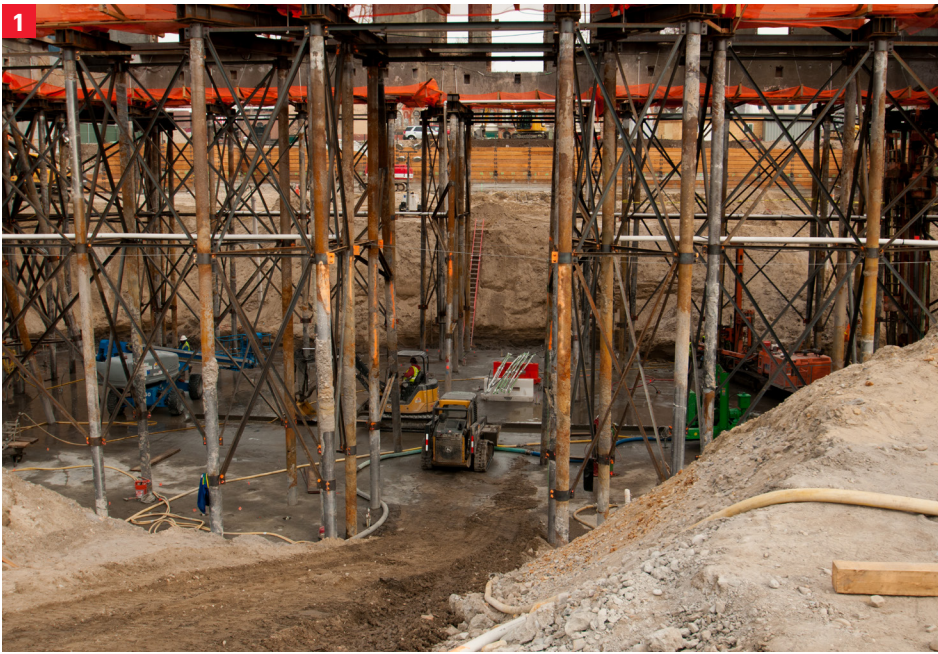
(1) Excavation with micropiles at Provo Temple (2) Micropiles at Provo Temple
