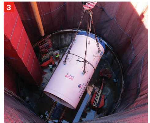
(1) Nicholson Superintendent and Foreman discussing TBM launch operation; (2 & 3) Lowering of Dorsey into the launch shaft at Virginia Key Central Wastewater Treatment Plant
