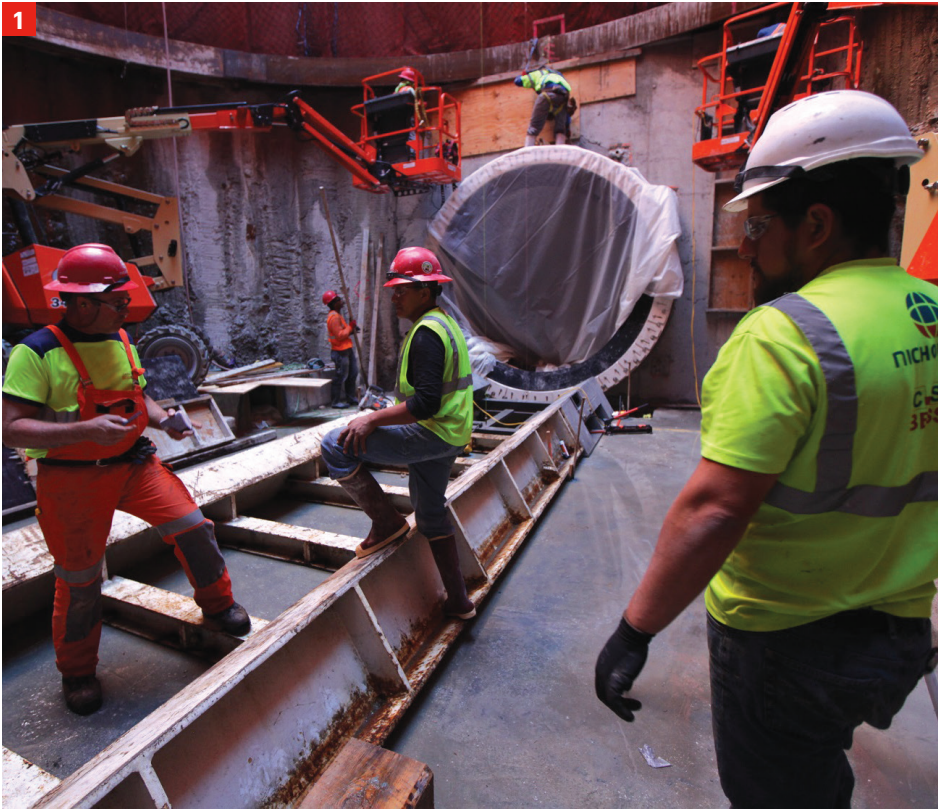
(1) Nicholson Superintendent and Foreman discussing TBM launch operation; (2 & 3) Lowering of Dorsey into the launch shaft at Virginia Key Central Wastewater Treatment Plant
