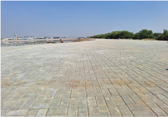
Road works in progress
