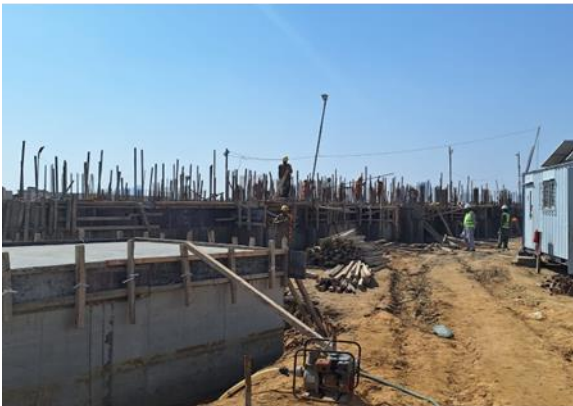
Ground Floor perimeter Beams
