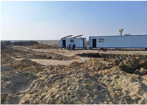
Mobilization on Site
