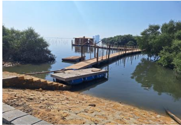
Walking Platform & Leaning center
