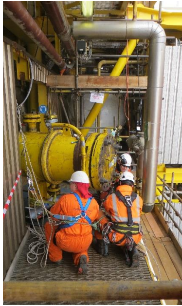
Photo: The Conbit rigging crew uses trolleys to move the separator outwards
