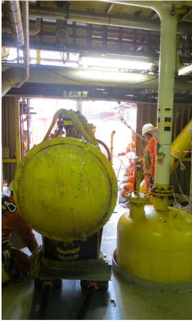
Photo: The Conbit rigging crew uses trolleys to move the separator outwards
