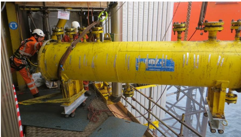
Photo: Bringing vital equipment overboard is a job for specialists
